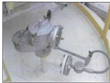
Pressure Vacuum Relief Valve
